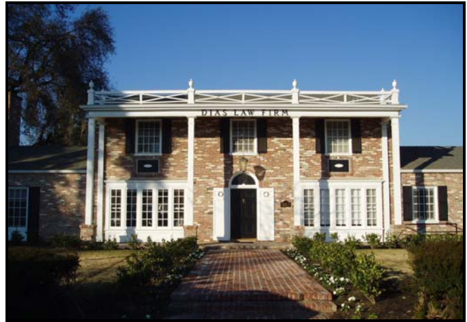
The Dias Law Firm moved to Grangeville Boulevard after refurbishing the property
